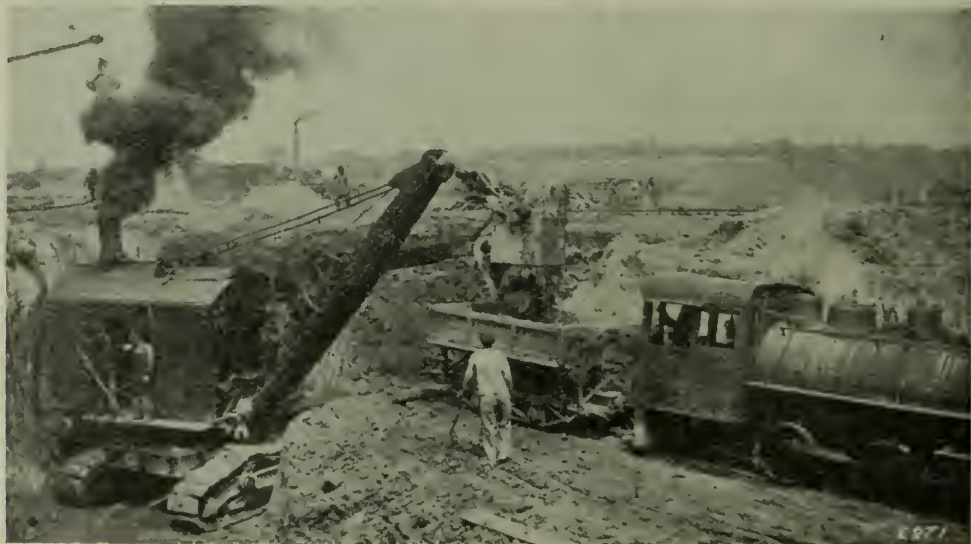
FIG. 10. STEAM SHOVEL WITH CATERPILLAR WHEELS.
